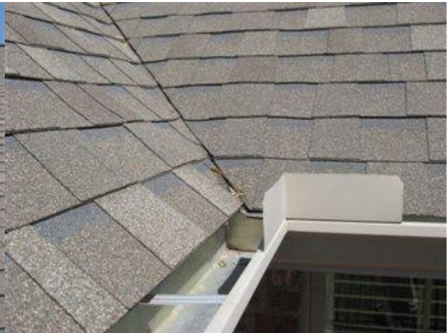
Photo 27 View of valley and guttering on west side
