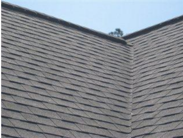
Photo 13 Close-up view of valley and ridge vents on the east side
