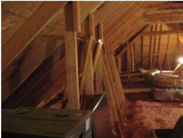
Photo 45 View of framing in attic
