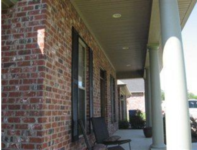
Photo 20 Recessed lights in front porch ceiling
