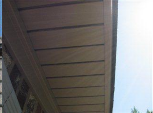
Photo 29 View of vinyl soffit covers with slots for ventilation
