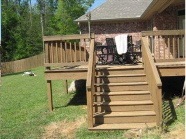
Photo 23 Deck stairs and railing
