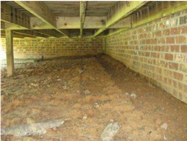
Photo 25 View of the grading underneath the deck
