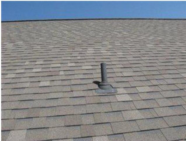
Photo 26 Sewer vent on the west side
