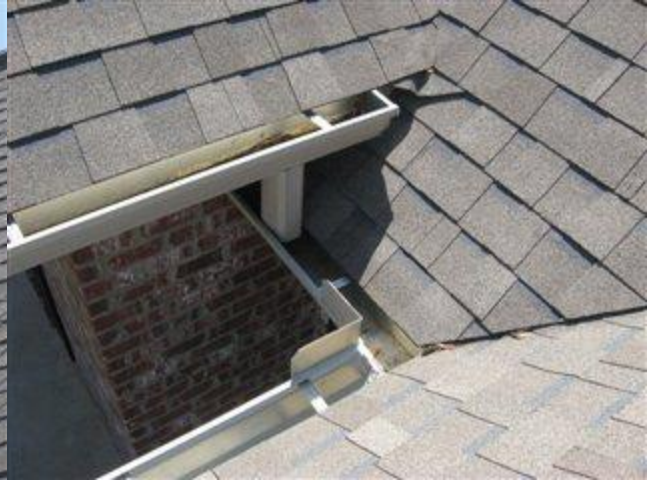
Photo 14 Overhead view of gutters and valley on the east side
