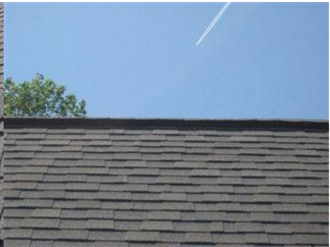
Photo 12 View of ridge vent caps from the east side
