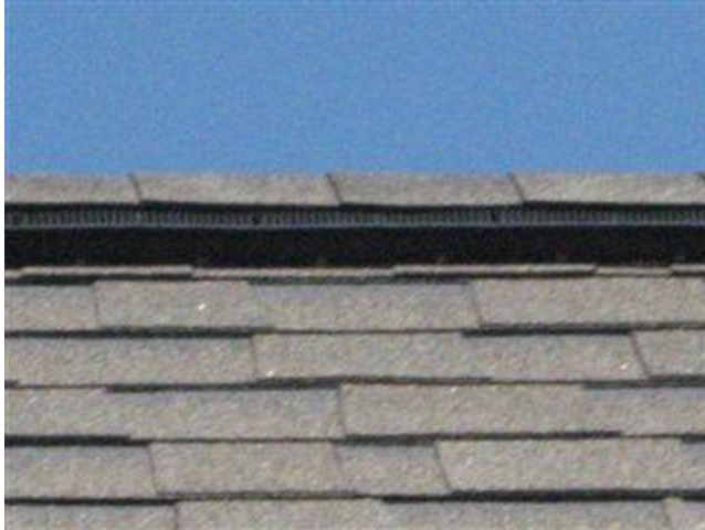
Photo 28 Close-up view of ridge vents from the west side
