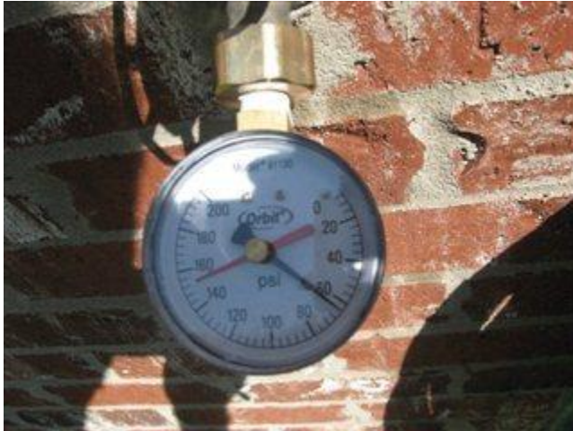
Photo 22 Water pressure measured at outside faucet
