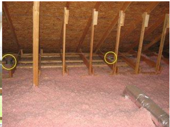
Photo 50 View from the attic of recessed can lights around the exterior
