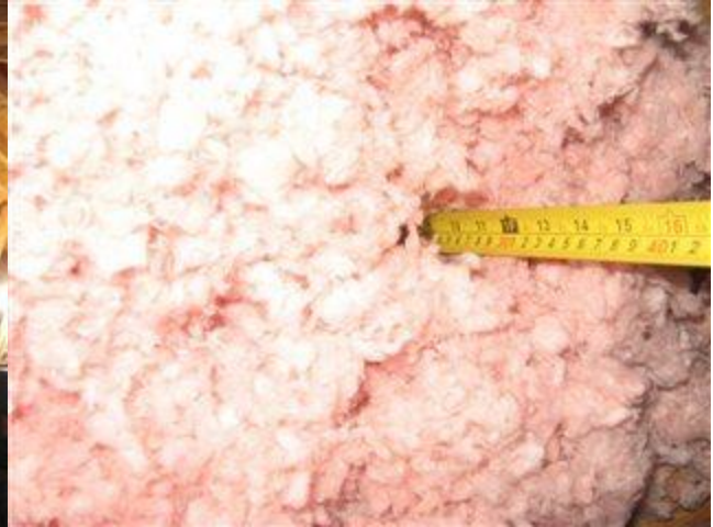
Photo 48 Showing depth of insulation measured at around 10" in accessible areas
