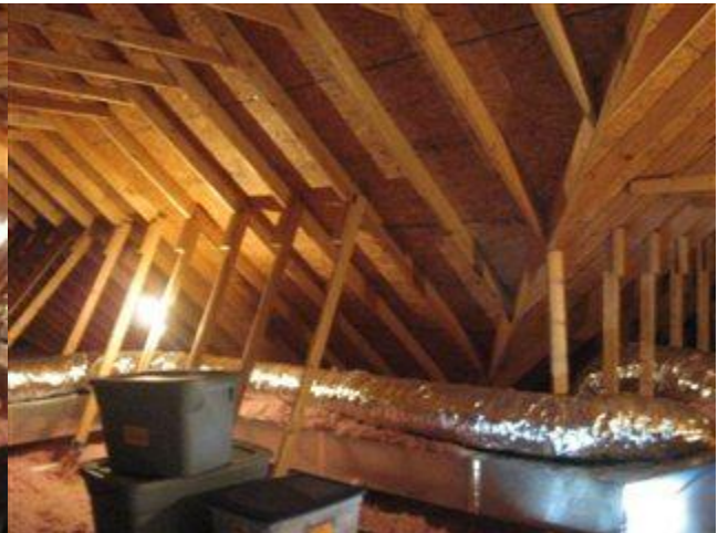
Photo 47 View of framing in attic
