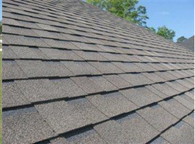
Photo 10 Architectural shingles on the east side with no defects noted
