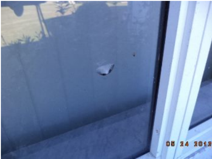
Window glass cracked. The fixed glass window at the left side toward the back of the house appears to have been hit with a small projectile and is damaged.
