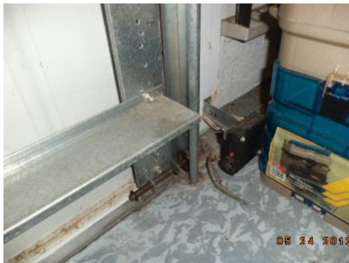
Garage vehicle door auto- reverse is inoperable on the one car garage door
