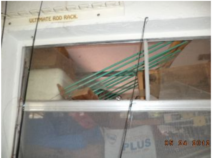
Window glass broken in between the existing garage and the garage addition on the interior. It is recommended to remove the broken glass for safety.
